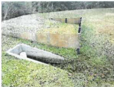
Overflow weir, skimmer and orifice (2018)
