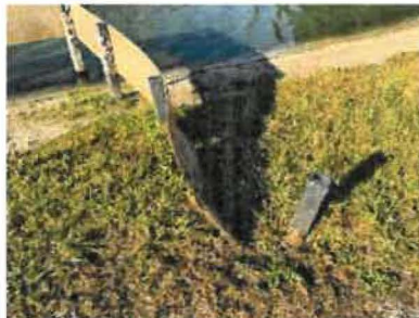
Damaged corner of skimmer (2018)
