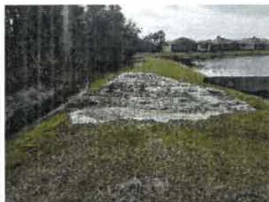
Overflow weir and spreader swale (2018)
