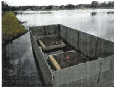
Control Structure Grates and skimmer (2018)
