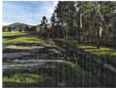
Overflow weir and spreader swale (2016)
