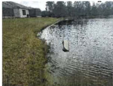
Inflow pipe #2 end section with shoreline erosion (2018)
