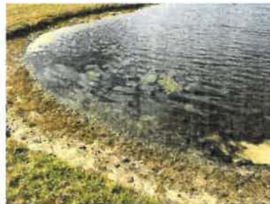
Signs of erosion and algae growth (2018)
