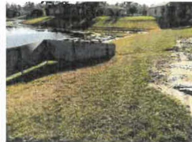
Missing section of skimmer (2018)
