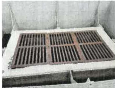
Control Structure Grate (2018)
