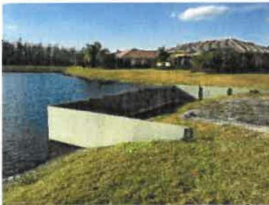
East overflow weir and skimmer (2018)
