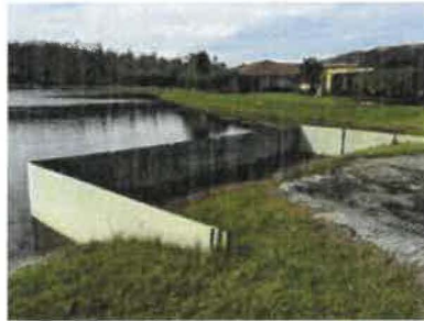
East overflow weir and Skimmer (2016)
