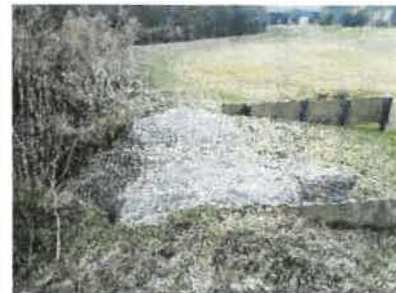
Overflow weir, skimmer and spreader swale (2018)
