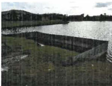
East overflow weir and skimmer (2018)
