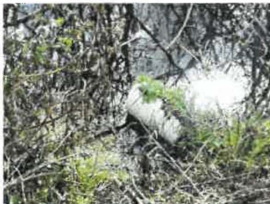
Pipe from orifice outflow into spreader swale (2018)
