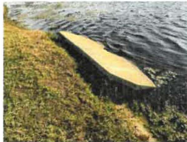
Inflow pipe end section with signs of shoreline erosion (2018)
