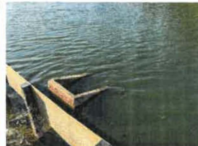
Orifice under water (2018)
