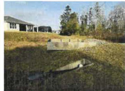
Overflow weir, skimmer and orifice (2018)
