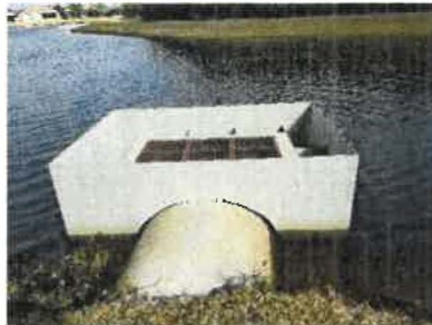
Control Structure and skimmer (2018)
