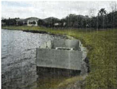
Control Structure and skimmer (2018)
