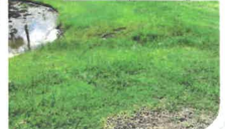
Minor pond bank erosion – Could benefit from drainage.
