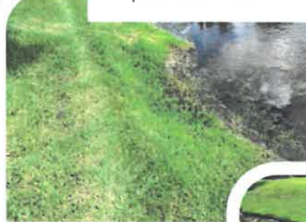
Minor pond bank erosion
