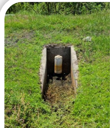
Figure 1 - Cleared bleeder Pipe
