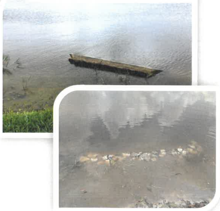
Figure 4 - Erosion behind MES on Pond 2
