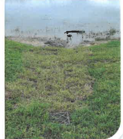
Erosion repaired with drain added to prevent future erosion.
