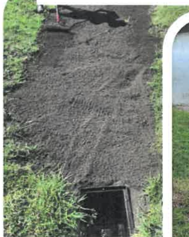
Grading bank and adding drain.
