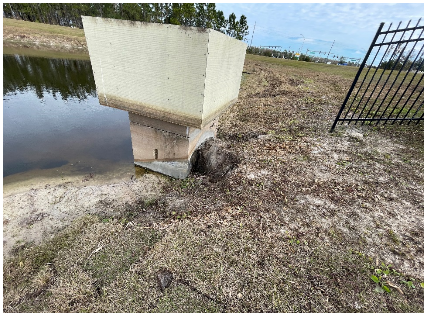
Exhibit 2 – Erosion behind structure on the east side
