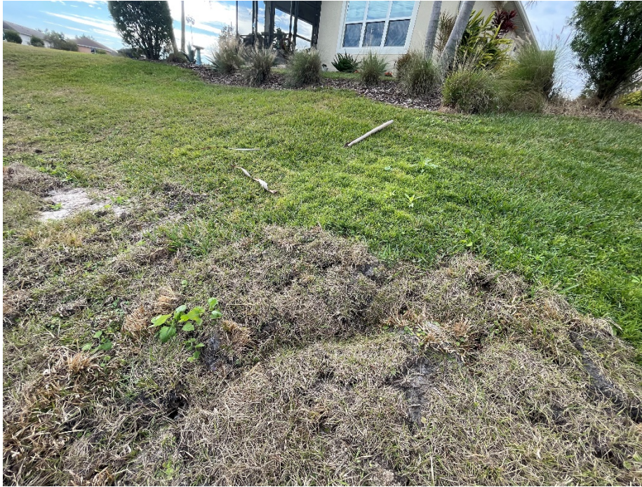
Exhibit 7 Gully in newly placed sod on the southern edge of the pond closest to Solivita Blvd.
