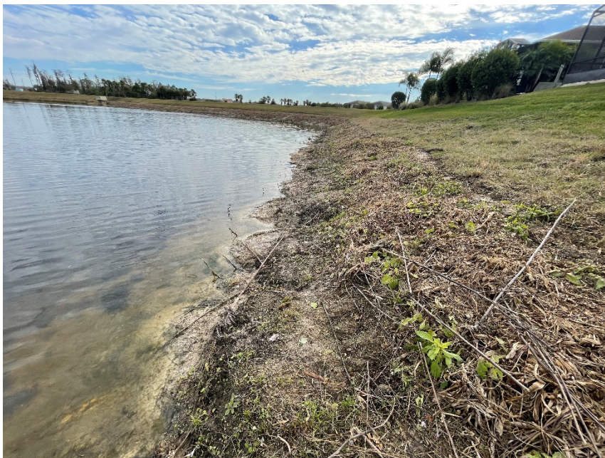
Exhibit 4 View looking east along the south pond bank. Netting exists of original sod about 3 ft above water line
