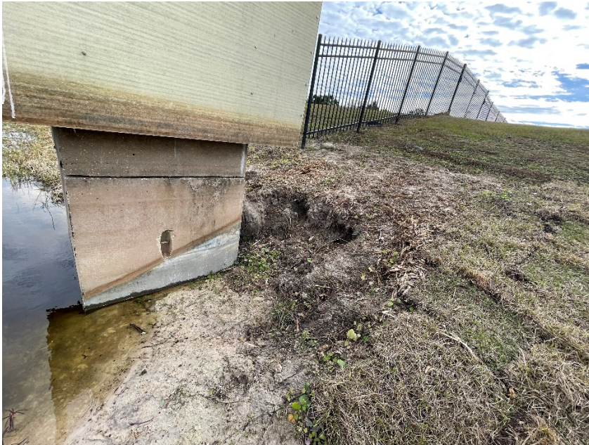
Exhibit 1 – Erosion around structure on the east side
